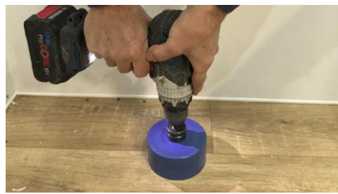
Fig. 8.2: Drill a \phi 102-105mm hole
