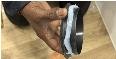
Fig. 8.3: Apply Silicon Sealant
