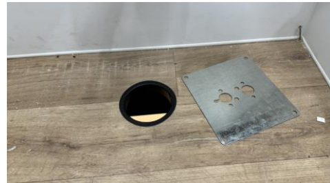
Fig. 8.4: Insert the metal ring
